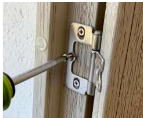
Final fix of screw in shutter hinge
