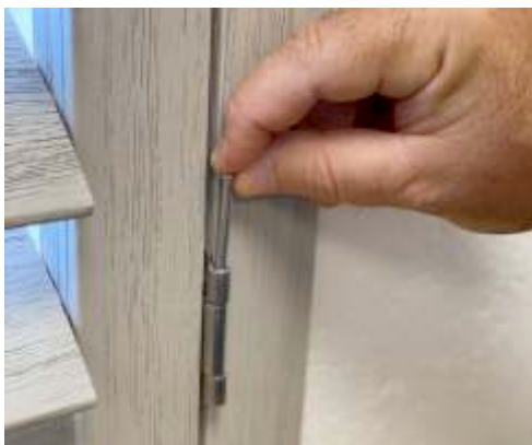
2 parts of hinge coming together with drop pin going in
